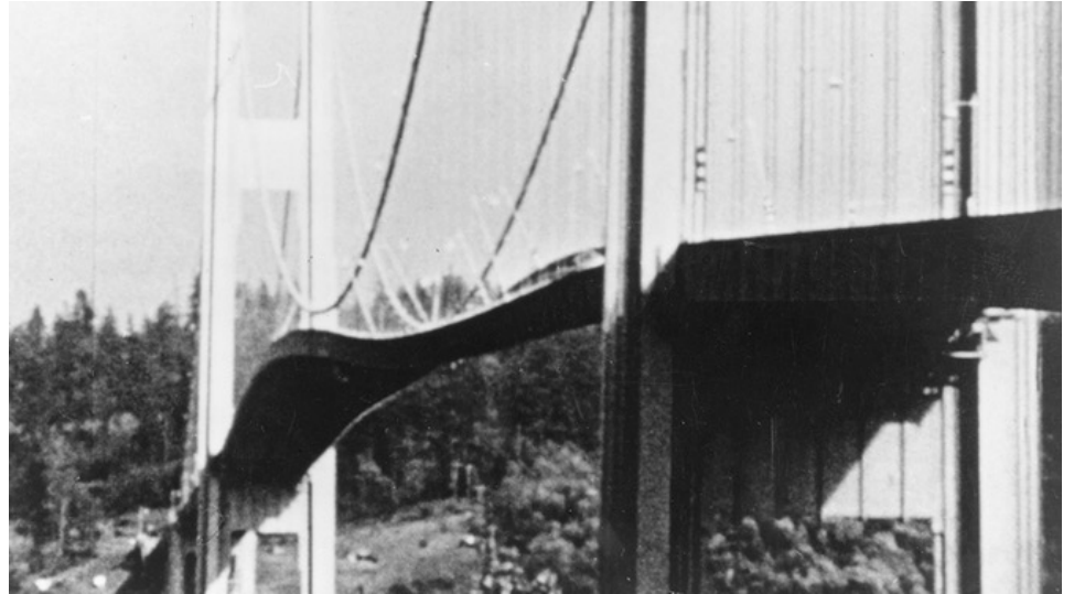
Collapse of newly opened Tacoma Narrows Bridge on November 7, 1940
